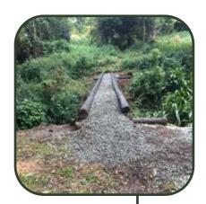
A bridge has been constructed over the stream utilising recycled street poles and 19mm stone. We have procured a brush cutter and the trail pathway will be cut along the contours of the Conservancy Park soon. The trail will provide access to walkers and bird watchers, and also facilitate ease of access for IAP maintenance.
